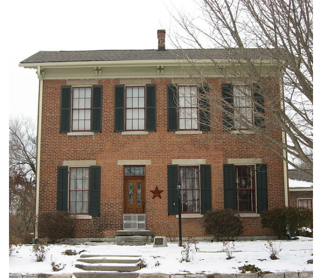
Cole-Evans House, built circa 1830s is a historic home featuring Greek Revival architecture
